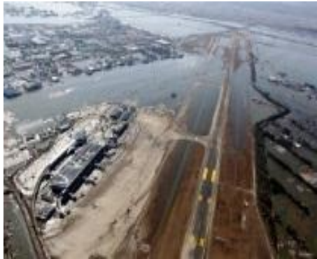
Drowned runways of Sendai Airport
