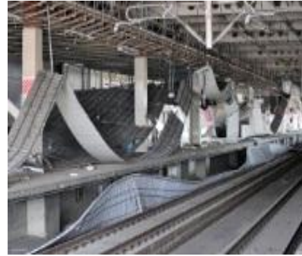
Collapsed roofs of Sendai station
