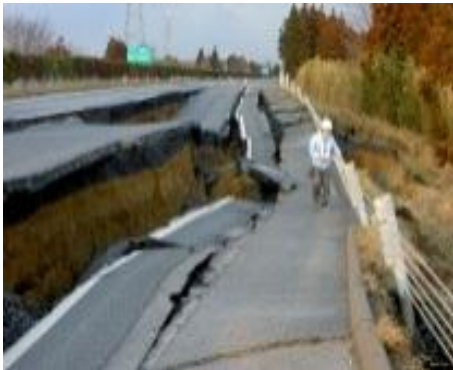
Subsided Joban Expressway
