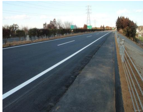
Restored Joban Expressway (March 17, 2011)
